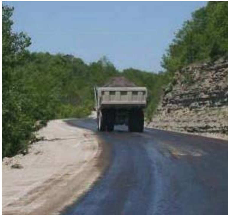
Treated road does not create coal dust.
